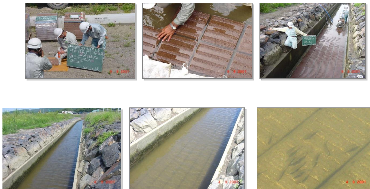
Fig. 3. Construction and Placement of EBB in river
